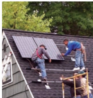
The 1140 watt system shown above was installed by a crew of three in less than a day.
