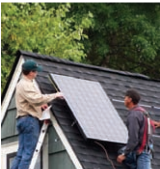
The 1140 watt system shown above was installed by a crew of three in less than a day.
