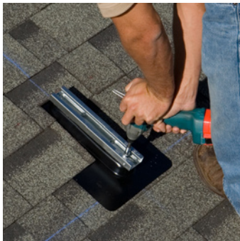
The adjustable slider assemblies make it easier to achieve straight rail alignment
