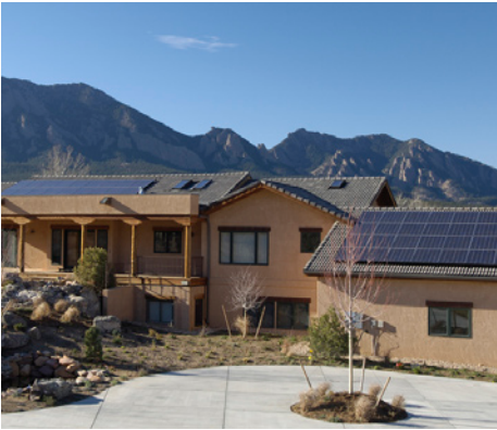
This residence is powered by a 8.3 kW grid-tied solar system with battery backup
