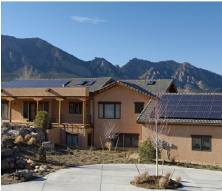
This residence is powered by a 8.3 kW grid-tied solar system with battery backup
